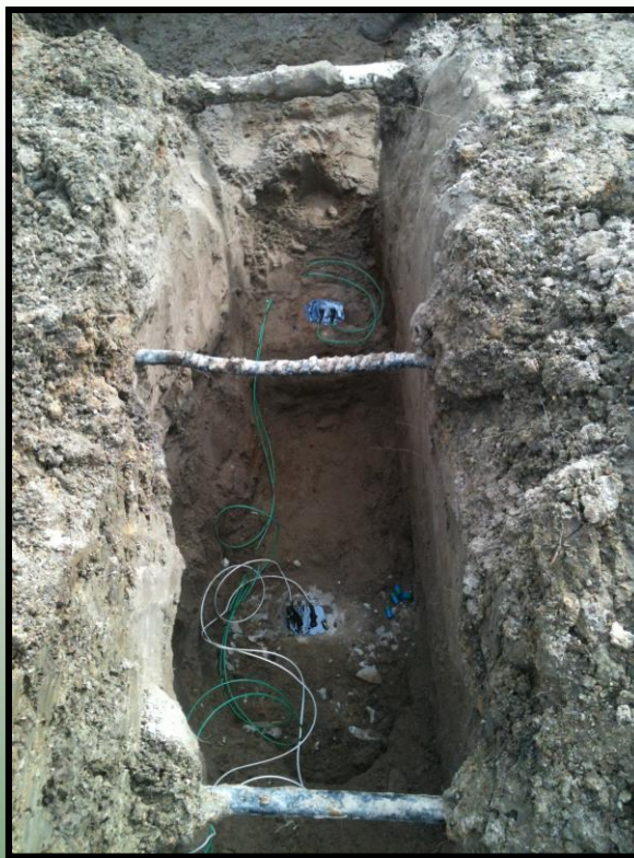
Typical test wire connections at casing.
