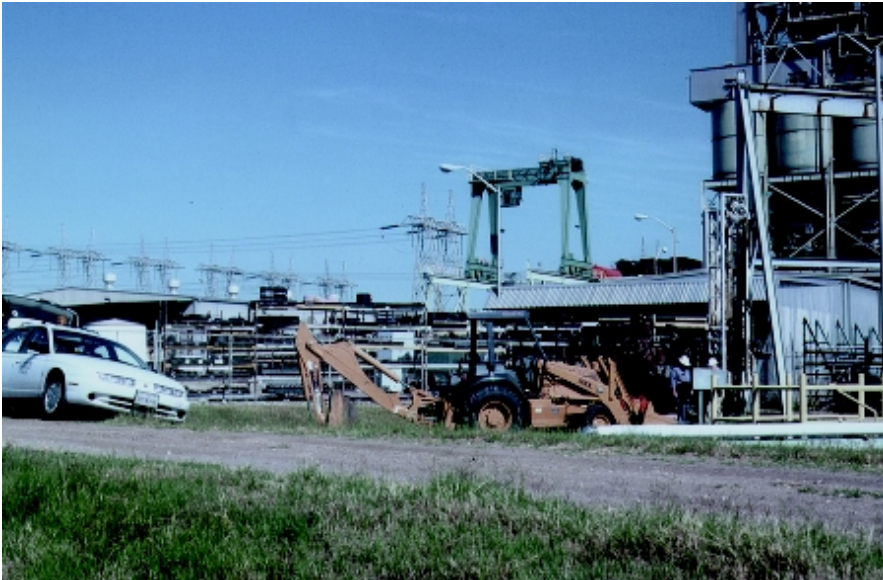
Typical construction activity, not related to CP work. Such construction may damage buried CP components.
