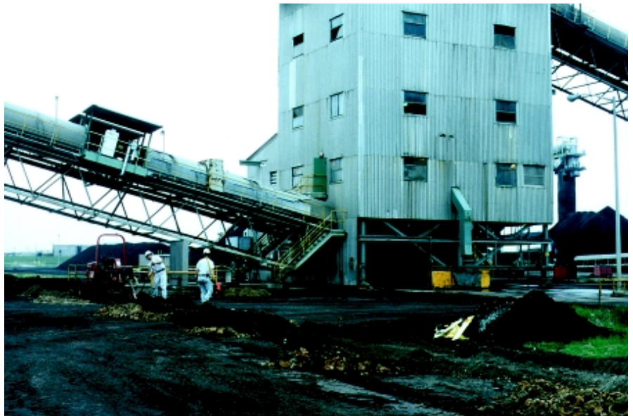
Repairs being made on a CP groundbed at the generating station.
