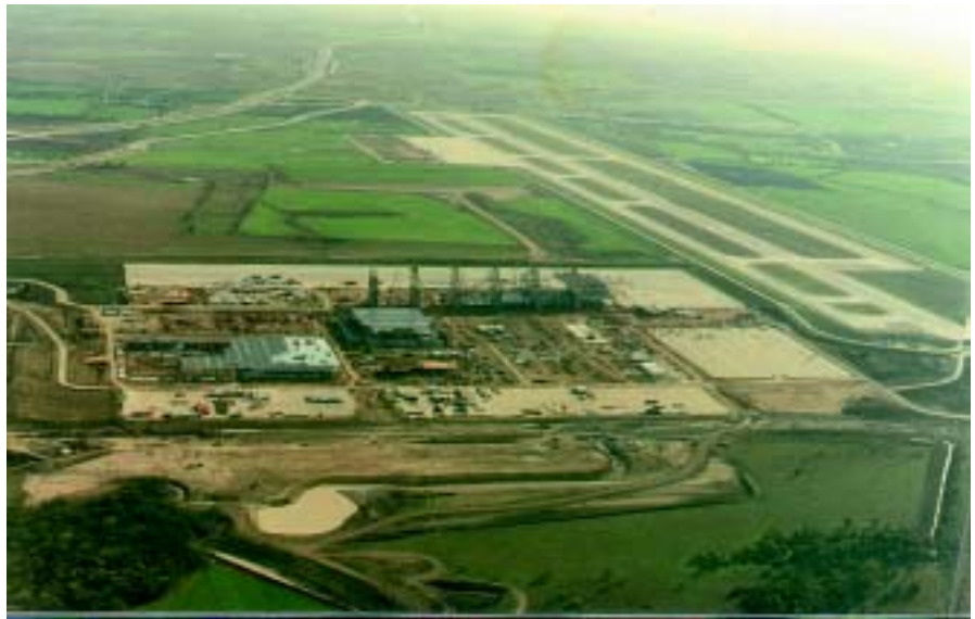
The American Airlines Alliance Maintenance and Engineering Base under construction.
